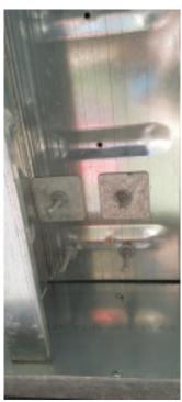
Figure 4. The author modified the original Paverdeck stair framing design, beefing it up with boxed galvanized LGS stringers and joists (top left), and forming the treads and risers with Paverdeck pans (above left). The through-bolts that attached the posts through the stone treads to the Paverdeck pans were backed with large washers (above right).
