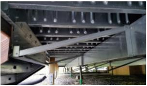
Figure 2. The LGS joists on the upper deck hang from galvanized rim track with preformed, prepunched tabs at standard spacings (top). Diagonal bracing was installed on the lower deck to solve a pesky vibration problem in the steel deck framing (above).
