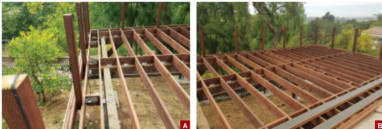
Figure 4. The deck posts were 45 inches high and through-bolted to the double rim joist with SST DTT2Z anchors, reinforced with plenty of blocking (A). The posts were located on 4-foot centers because of the shallow 2x8 joists (B).
