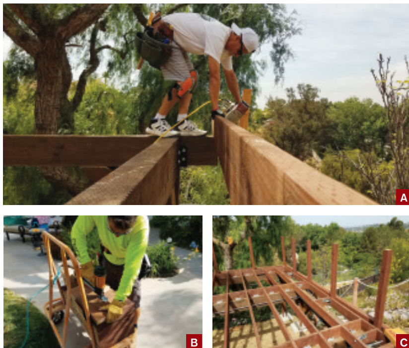
Figure 3. Even though most of the deck is elevated, 2x8 joists were needed to avoid having a tall step up onto the deck from the adjacent patio (A). Joist blocks were pre-fitted with SST A35 framing angles (B), then fastened to the beams to help limit lateral movement and to provide some uplift value (C).
