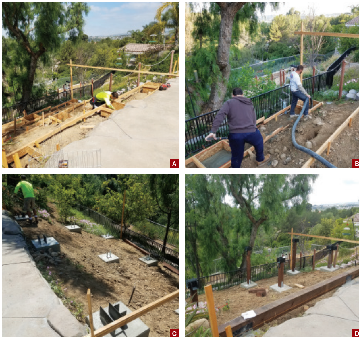
Figure 1. The freestanding deck is located on a steep slope and just one step up from a hardscaped pool surround (A). Nine 2-foot-square-by-30-inch-deep footing forms were filled with 4,500-psi concrete (B); metal hardware to connect the framing to the footings was embedded in the concrete during the pour (C). The upper three footings support a continuous 6x12 PT beam; the other footings support 6x6 posts (D).
