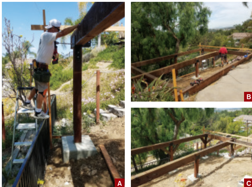
Figure 2. Beams were bolted to the black-painted brackets with \frac{5}{8} -inch-diameter HDG bolts (A). The carrying beams were tied together with perpendicular perimeter beams to reinforce the frame against seismic loads (B). The frame was also reinforced in both directions with knee braces that were fastened to the beams and columns with \frac{1}{2} -inch-diameter HDG all-thread rod (C).
