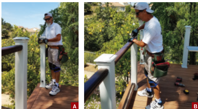
Figure 7. The author used a laser distance measurer to determine guardrail lengths (A). The Trex railing is 42 inches high, to meet California code requirements (B).
