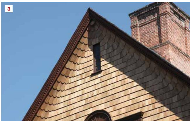
A photo from 1906 shows Naumkeag, in Stockbridge, Mass., with the original decorative shingling (1). Elaborate staging allows the crew to reach the gable peaks (2). The restoration crew replicated the curved scalloped shingles along the gable eaves (3).
