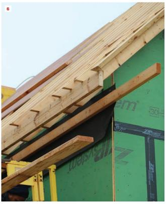
The crew installs all the common rafters before beginning to frame the cornice (5). The subfascia fits into the notch cut into the rafters, and the soffit ledger attaches to the wall over a layer of 30-lb. felt paper (6). Blocking next to each rafter spans between the subfascia and the ledger. The angled crown backer fits against the subfascia and the horizontal cut of the rafters (7). The backer is mitered at all inside and outside corners.
