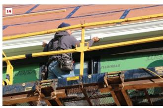
Using a gauging block to draw a line for the bottom of the crown molding ensures its accurate placement (11). Because the PVC crown stock is so floppy, the crew cuts it on the flat, using the detents on a chop saw (12). The crew then aligns the crown with the gauge lines and nails the pieces into place (13). The gauge block is used again, this time to ensure that the fascia reveal is even all the way around the house (14).
