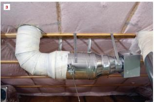
Here's a closer look at the home's air intake ports: a fanpowered inlet that supplies continuous fresh air (2) and a makeup-air inlet with a weighted passive damper that opens only if exhaust vent fans depressurize the house (3).
