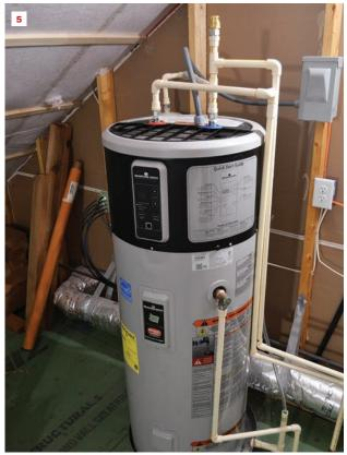
A large jump duct in the attic floor allows free airflow between each bedroom and the buffer space for pressure relief (4). A heat-pump water heater (5) recovers latent heat from the indrawn air, helping to dehumidify the space as it heats water.
