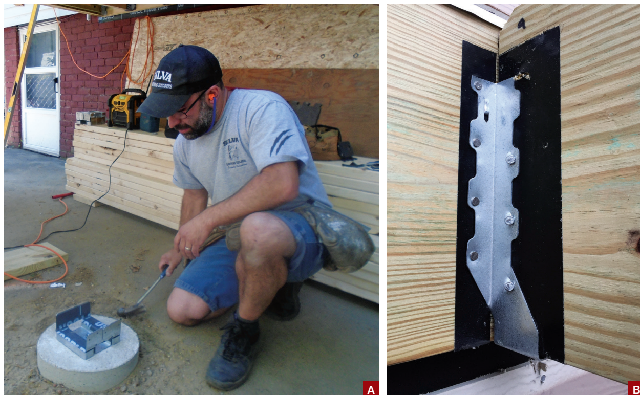
Figure 5. Covering the top surfaces of a galvanized post base with strips of self-adhesive membrane before setting the post in place helps to isolate the metal connector from the corrosive effects of pressure-treated lumber (A). Though newer PT formulations aren't as corrosive as ACQ-treated lumber, many builders still wrap joist ends with self-adhesive flashing tape prior to hardware installation (B).
