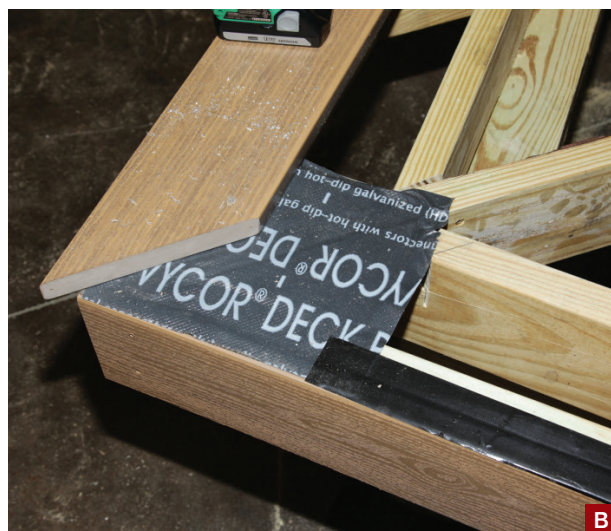
Figure 2. Cuts and end-grain in PT lumber should always be field-treated with a copper naphthenate-based preservative (A). Many builders use self-adhesive membranes in various widths to protect deck framing from moisture. Here, narrow tape covers the gap between the fascia and rim, while wider pieces of membrane protect corners and doubled framing (B).
