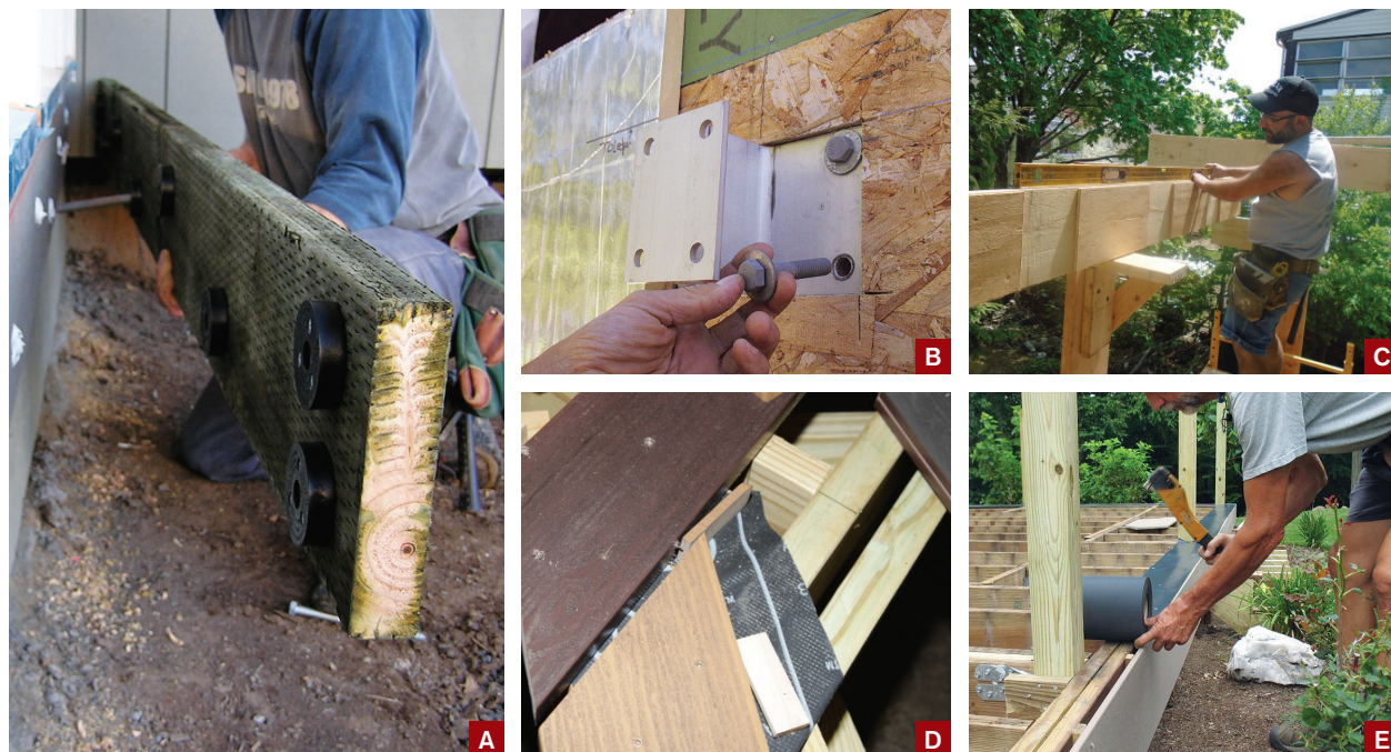
Figure 4. Deck2Wall's code-approved spacers are fastened to the back of the ledger to promote drainage between the house and ledger (A). Made of solid aluminum, Maine Deck Brackets also create a structurally sound method of keeping water away from the house and ledger (B). PT plywood or PVC spacers can be used to create drainage gaps between the 2-by layers of a built-up beam, preventing water from being trapped between doubled framing members (C). Gapping miters at intersecting deck boards will allow water to quickly drain away from vulnerable end cuts (D). PT spacers between the fascia and framing and a membrane cap over the gap will minimize potential water damage to the rim joists (E).
