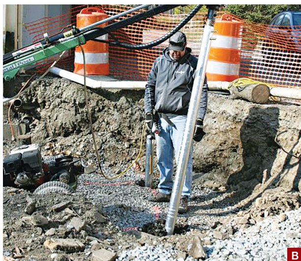
Figure 1. A pair of 1/2-inch rebar rods embedded in the fresh concrete will tie the pier to the expanded footing below the cardboard form, creating a more stable foundation (A). Helical piers can be installed in any weather, have a higher load capacity than concrete, and require less cleanup (B). Though more expensive than concrete piers, they are helpful in poor soil conditions, or where frost heave is a concern.
