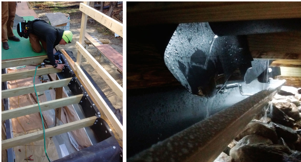
Figure 4. To protect the rim joist, the author makes scuppers out of the scalloped pieces that were cut from the membrane (above left). Water flowing off the membrane will be deflected by the scuppers into the gutter (above right).
