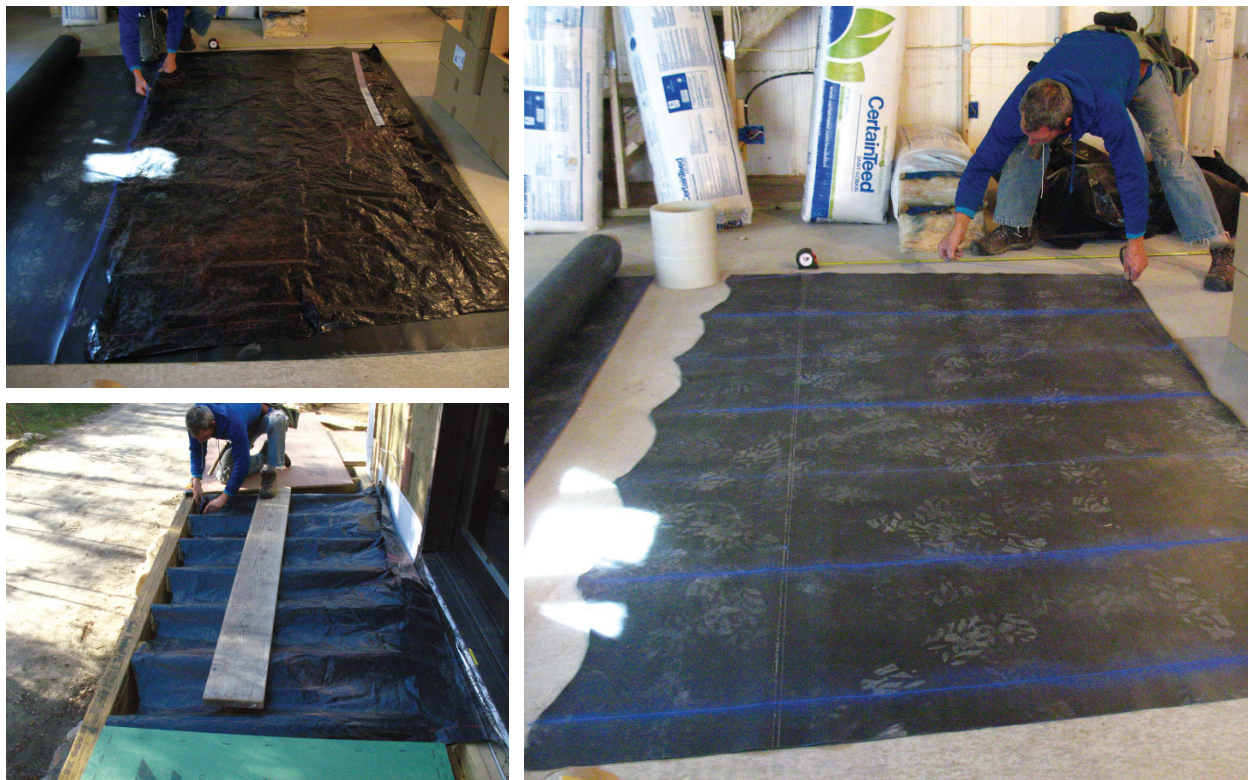
Figure 3. Using a piece of black plastic (an old tarp could also be used), the author makes a template for the membrane (top left). Referring to the dimensions in Figure 2, he snaps chalk lines for the centerline and joists onto the template, then drapes the template over the deck framing so that the chalk lines are aligned with the joists (above left). He trims the template to fit, then uses the template as a pattern for cutting out the EPDM membrane (above right).
