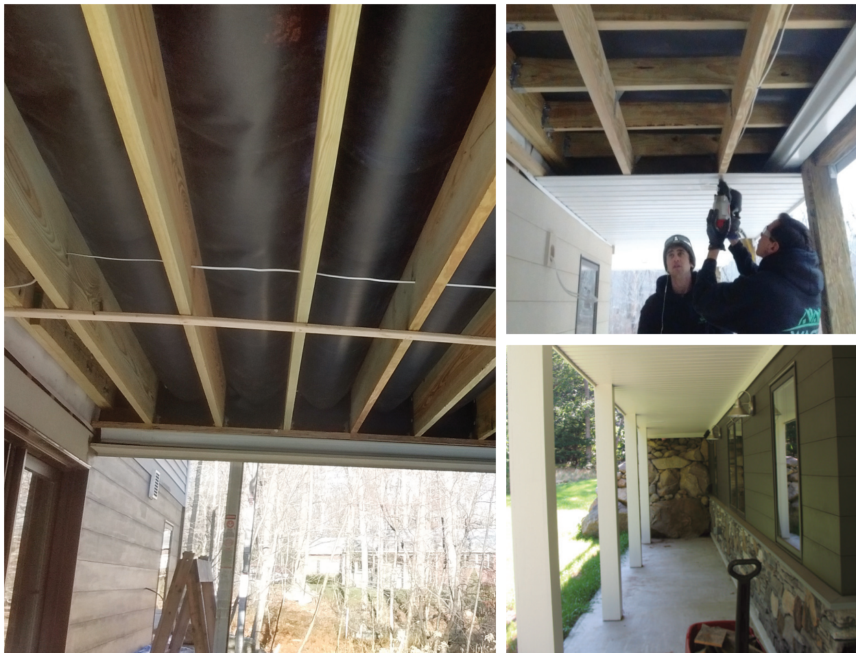
Figure 7. To finish the system, the gutter can be boxed in and the bottom of the joists covered with vinyl soffit (above left). Another option is to install a dropped beadboard ceiling that covers the gutter and rim joist (top right). Though not required, a ceiling applied to the bottom of the joists gives the space a finished look (above right).
