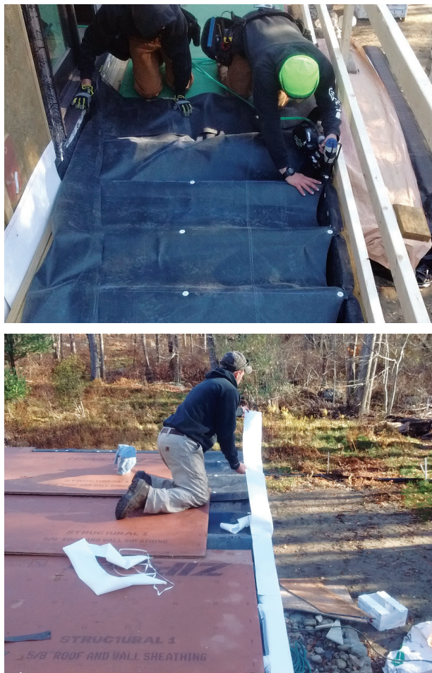
Figure 5. Working from the center, workers use cap fasteners to attach the membrane to the joists (top). A strip of self-adhering flashing tape covers the joints between the scuppers and protects the rim joist (above).
