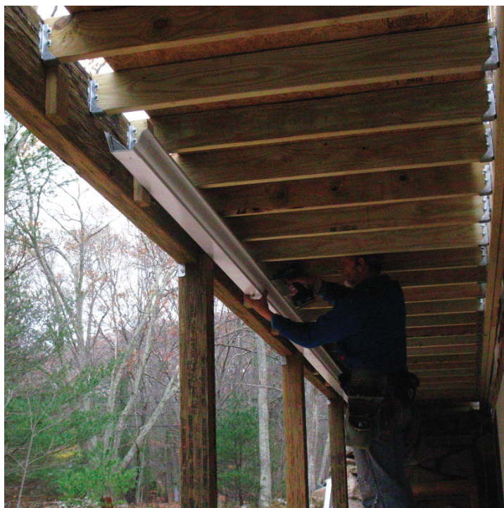
Figure 1. Water from the under-deck drain system is collected by a standard “K”-style aluminum gutter. When installing a system, the author typically oversizes the rim joist to accommodate the gutter.
