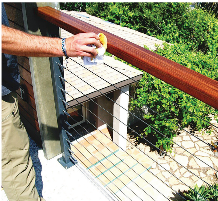
Figure 7. Routine cleaning and maintenance with a penetrating oil finish is needed to keep the ipe top rail looking good in a marine environment.
