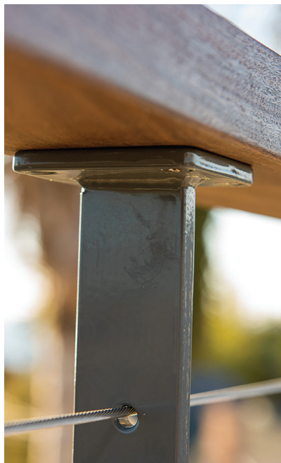
Figure 4. By upgrading from a \frac{3}{4} -inch-thick to a full-2x4 ipe top rail, the author was able to eliminate the metal subrail typically used with aluminum and lighter-gauge stainless steel rail systems.
