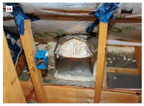
Because the home needed new roofing shingles, and because some sheathing was damaged and needed replacing, the owners decided to repair the system from outside (11). But some spaces were also accessible from inside. A small attic space was insulated from inside (12). That ceiling got a smart vapor-control membrane (13), and the crew sealed a bath fan (14).
