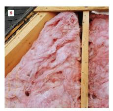
Originally a simple raised ranch, this home had been remodeled with complex architectural details (1, 2), which made adding to the roof's thickness impractical. The shingle roof needed replacement, and there was mold and rot in some areas of roof sheathing (3, 4). Existing fiberglass insulation (5) was compromised by installation gaps and voids, as well as mouse tunnels.
