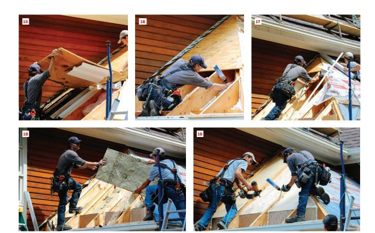
Working from outside, the crew removed the existing sheathing (15), filled gaps between the ceiling and the rafters (16), nailed cleats to the sides of the rafters (17), and insulated the cavities with Roxul mineral wool (18). They protected the insulation with lauan plywood (19), also creating an air space to help cool and dry the roof system.
