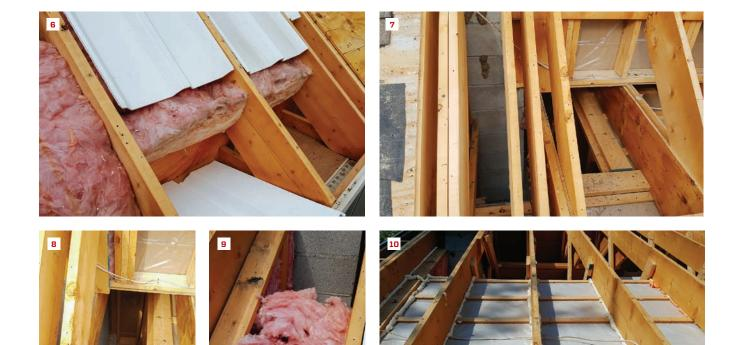
Existing fiberglass batts in the rafter bays were exposed to wind-washing at the eaves (6). Complicated existing framing around the chimney, an older original roof that had been left in place, and the later belvedere addition had created a maze of interconnected air bypasses (7, 8, 9). For this rehab, the existing ceiling (10) was left in place, and the roof upgraded from above.
