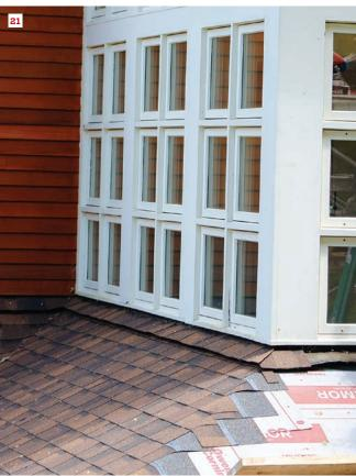
Where roofs abutted walls, the crew installed Cor-A-Vent Roof-2-Wall vent to allow air in the rafter vent channels to exit the system (20, 21). Ridge vents (using Owens Corning VentSure; not shown) were also installed where feasible. The solution chosen allowed the repair to take place without any disruption to the existing windows.
