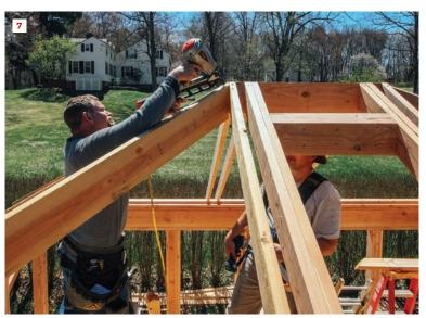
To install the hip rafter, set the top end into the corner between the two king commons and tap it down until the shoulders are flush with the tops of the adjacent rafters (5). Align the edge of the seat cut with the layout line on the plates and toenail it from both sides (6). Fasten the top through the king commons if accessible or directly through the top (7).
