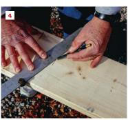
Lay out plumb cuts for the top of the hip rafter (1), and make the cuts with the saw blade set at  $45^{\circ}$  (2). Swing an arc at the measured length of the rafter (3), and then mark the HAP along an intersecting plumb line (4). Using the ruler on the framing square, the  $4^{3}$ /s-inch HAP is marked at  $10^{3}$ /s inches. These steps are also shown in the illustration below.
