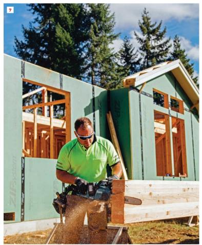
Only recently introduced, DeWalt's in-line saw (5) is well-balanced and cuts faster than, though not as deep as, the Makita. The last surviving corded saw on Uhler's site is the 10-inch Big Foot saw (6). It's only used these days for finish beam cuts. Rough cuts on large beams are easily handled by a cordless chain saw, such as this 36V (dual 18V) Makita (7).
