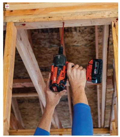
The high torque and long runtime of the Makita XPHO7T (8) have allowed it to replace all the author's corded drills for all drilling and hole-cutting tasks. For driving many fasteners, DeWalt's 20V Max drill/driver (9) serves well, but for long structural fasteners, the author needs the extra power of an impact driver, such as the Milwaukee M18 (10).
