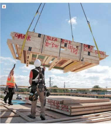
BMC's ReadyFrame provides lumber packages with precut plates, jack studs, headers, and cripples. Plates come printed with each wall layout (1), so framers only have to grab precut studs from a pile and assemble the wall; no layout or cutting required. HomeTechnology is making inroads to North American housing markets with fully assembled floors, walls (2), and roofs (3).
