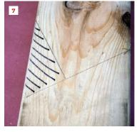
Rafter stock. I start by selecting material that's as straight and free of twists as possible. Even good lumber usually has a bit of a crown, so I sight down the edge of the material (1), and place a mark pointing to the edge where the crown faces up. We will install the rafters with crowns facing up, so I place that side towards me on a bench or sawhorses.
