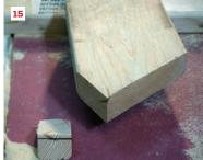
Tail cut. In our example, the roof has a 9-inch overhang as measured on a level plane from the building (see Roof Plan, page 13). I lay this out by measuring horizontally across the rafter (8) from the birdsmouth shoulder. (It's not shown, but you may want to use a square to make sure you are pulling the tape square to the birdsmouth shoulder.) I mark a plumb line here using the layout square, the same way I did for the top cut and for the shoulder of the birdsmouth.
