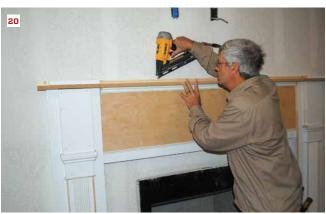
Mantel shelf. The author scribes the mantel shelf to the pilasters and panels (16), and then offsets the lines for the layers of molding. Initial cuts made on a table saw are finished with an oscillating cutter (17). A pieced-in layer of MDF adds thickness to the shelf (18). A straightedge ensures that the shelf is flat (19) before it's attached to the mantel below (20).
