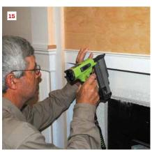
**Pilaster installation.** To position the pilasters, the author draws plumb lines beyond the code minimum clearance (10). Before securing attachment boards to the wall, he levels between them (11). He nails the pilasters to the boards (12) and the panel sections to the pilasters (13), then adds a built-up panel between the pilasters (14), trimming it to finish the plywood edge (15).
