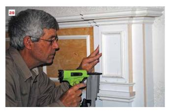
Creating the panels. Molding outlines on the flat surfaces create a paneled look. A spacer block positions the preassembled side pieces (25), which then rest on the block during installation (26). The center panel has inverted corners for added interest (27). At the pilasters, a horizontal bead of molding gives the panel a better proportion (28), and a rectangle of molding creates the pilaster panel (29).
