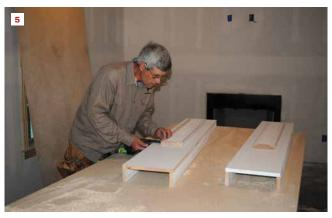
**Build the pilasters.** The pilasters that flank both sides of the firebox are designed to look like columns. The author screws and glues together U-shaped pieces that act as the foundation for the pilasters (1). A router with a flush trim bit evens out the edges (2). To simulate fluting, the author mounts reeded molding to 1-by boards (3). He adds small strips to the sides of the reeded boards (4) before mounting the boards to the pilaster foundations (5).
