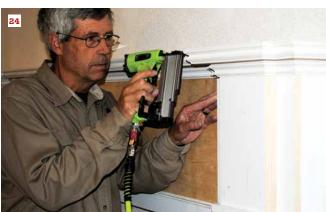
**Shelf trim.** Panel molding tops the pilasters below the mantel shelf. The author marks the length of each piece of molding in place (21), and then cuts it carefully on a miter saw using a stop (22). He then nails each piece onto the mantel (23). Another band of molding wraps around the edge of the mantel shelf, as well, following the contours of the pilaster below (24).
