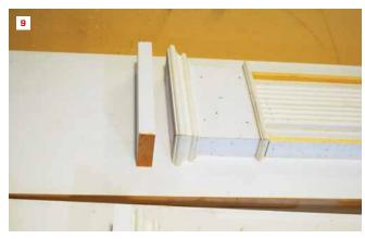
Bases and capitals. To complete the columned look, each reeded section receives a base and a capital. After finishing the bottom of the reeded section with a 1-by block, the author wraps the block with panel molding (6), below which he installs a U-shaped base (7). For the capitals, he installs smaller U-shaped pieces above the reeded sections (8) and then adds layers of molding and a block for the "top" of the column (9).
