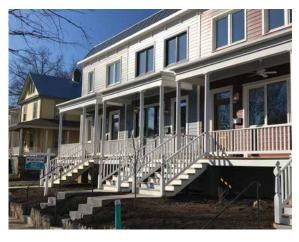
This high-performance townhouse project, although precertified as a Passive House building, didn't comply with Maryland's prescriptive energy code because some of the windows, chosen for a winter solar heating contribution, exceeded the state's maximum Solar Heat Gain Coefficient (SHGC).
