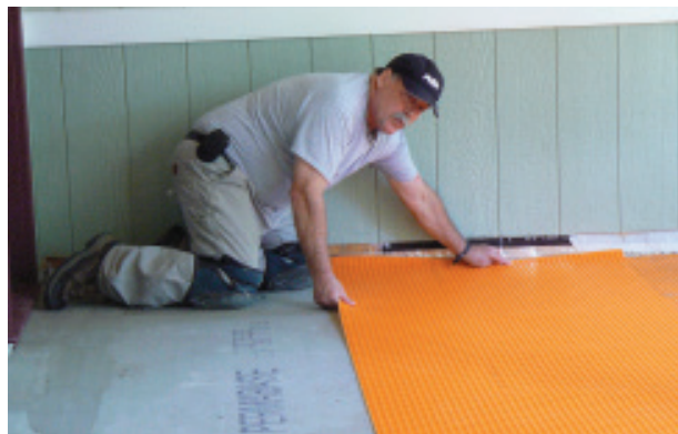
Figure 2. Before installing the Schluter-Ditra waterproofing membrane, the author cut and dry-fit all the pieces, marking their position on the floor with a pencil before rolling them back up.
