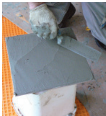
Figure 10. To ensure enough coverage over the waffled surface of the Schluter-Ditra membrane, the author also back-buttered every tile.
