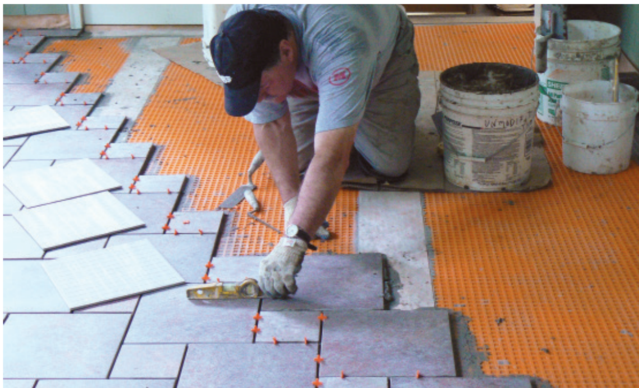
Figure 8. The author installed the porcelain tile in a pinwheel pattern, which required two different sizes of square tiles. Usually (but not always), the dimensions of one tile in this pattern are twice the dimensions of the other. In this case, the large tile was 11\frac{3}{4} inches square and the small tile was 5\frac{3}{4} inches square. With a \frac{1}{4} -inch mortar joint, the size of the increments for the layout ended up an even 12 inches and 6 inches.
