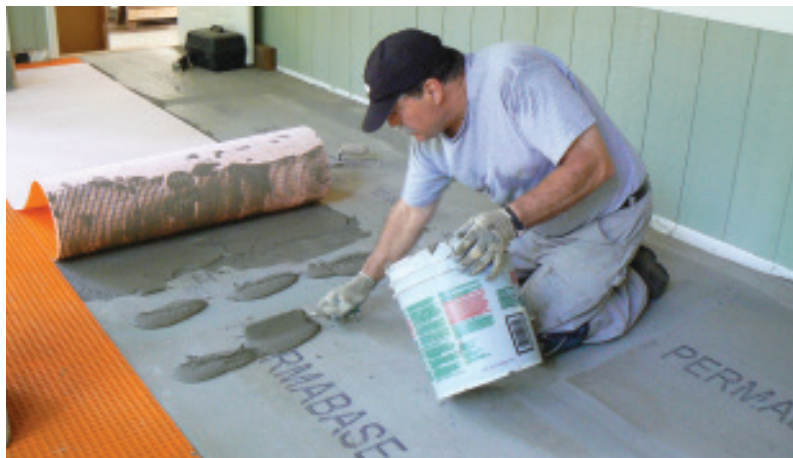
Figure 5. After embedding the first half of each strip of membrane in the thinset, the author rolled back the second half and repeated the process.
