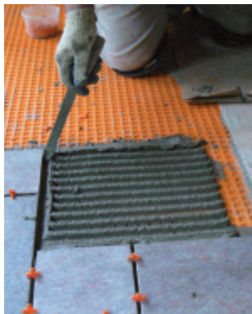
Figure 9. The author set the tile in unmodified thinset applied with a 1/2-inch-by-1/2-inch notched trowel.
