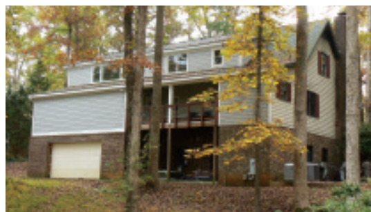
Figure 12. Even after four years of use, the porch floor looks as good as the day the tile was installed (top), with no signs of leakage under the porch (above).
