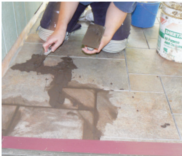
Figure 11. After the tile was set and the thinset had cured, sanded grout was used to fill the joints.
