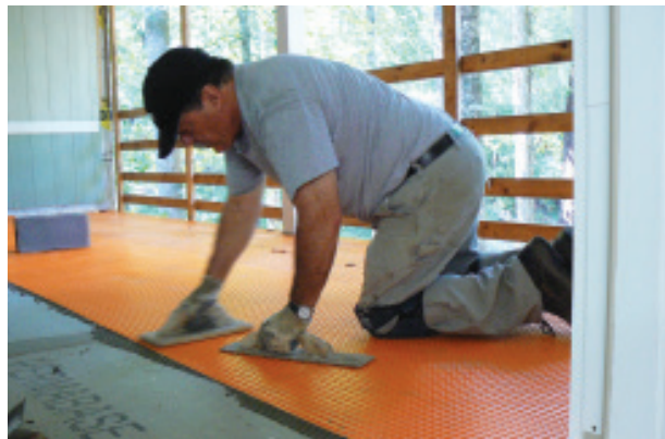
Figure 4. Wooden hand floats were used to press the membrane into the mud, working from the inside out to make it easier to avoid bubbles in the membrane.
