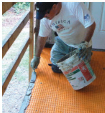
Figure 7. To finish the open edge of the porch, the author installed Schluter's Rondec-Step metal trim, first spreading a bed of thinset over the membrane (above left). After pressing the trim into place in the mud (above right), he placed a concrete block at each end to hold it in place while the mud set up.
