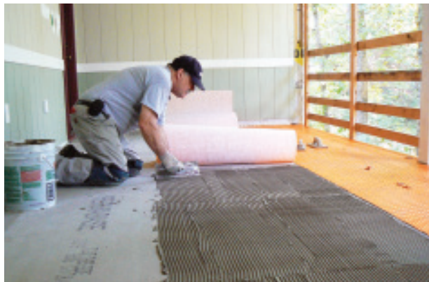
Figure 3. Working quickly, the author spread unmodified thinset mortar to the lines drawn on the floor, combed it with a ¼-inch notched trowel, then rolled the membrane back into place.
