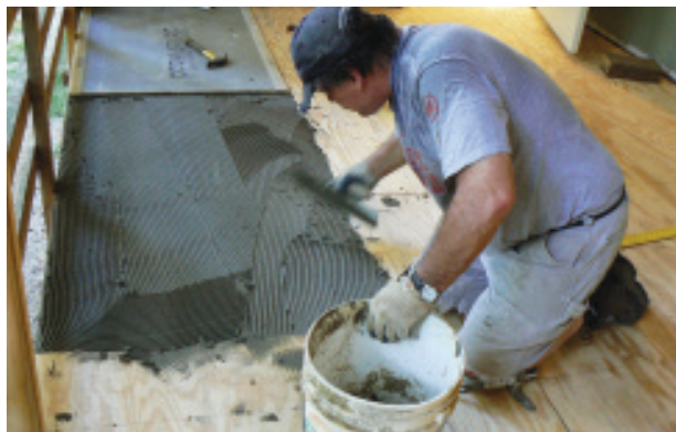
Figure 1. To prep the porch for tile, the author first installed a new plywood subfloor, followed by cement backerboard set in unmodified thinset adhesive and fastened to the subfloor with 1½-inch roofing nails.
