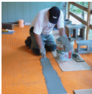
Figure 6. Membrane seams were taped with 5-inch Schluter Kerdi-Band embedded in unmodified thinset, in a process much like taping drywall (above left). Schluter Kerdi-Kereck preformed outside corners (above right) were used to flash the post-to-membrane intersection.
