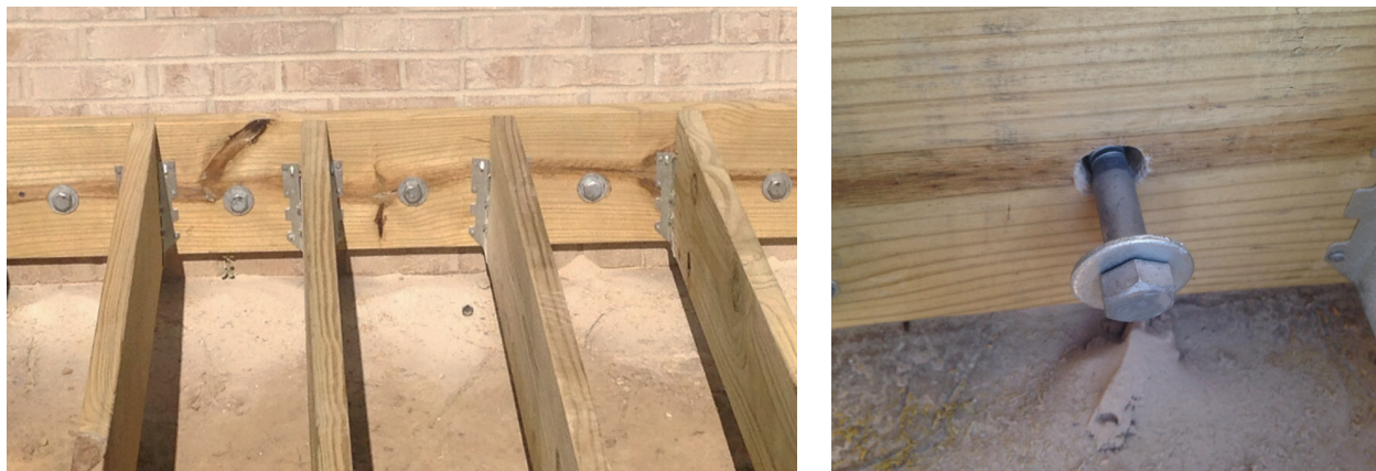
Figure 3. The ledger was fastened to the house rim joist with \frac{3}{4} -inch-by-8-inch galvanized lag screws installed on 12-inch centers (left). Oversized holes had to be bored through the brick veneer so that the ledger bolts wouldn't bear on the brick (right).
