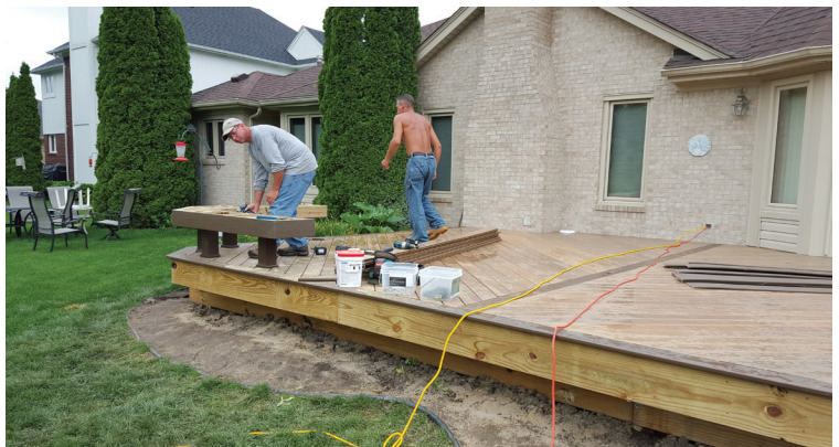
Figure 7. Blocking installed around the perimeter of the frame (left) supports the picture-frame detail used to finish the decking. A contrasting seam board in the middle of the deck highlights the diagonal decking (below). The deck has a tiered fascia detail, which makes the edge of the deck appear narrower (bottom).
