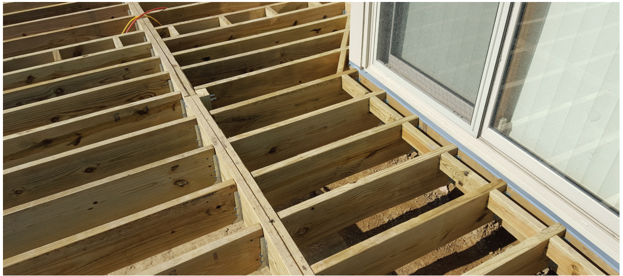
Figure 5. Siding and trim had to be removed from the cantilevered bay before this section of the ledger was installed. Deck loads here are supported primarily by the flush beam, with the cantilever ledger serving mainly for lateral attachment. Note the blocking, which eliminates the need to fasten the decking to the ledger through the L-flashing.
