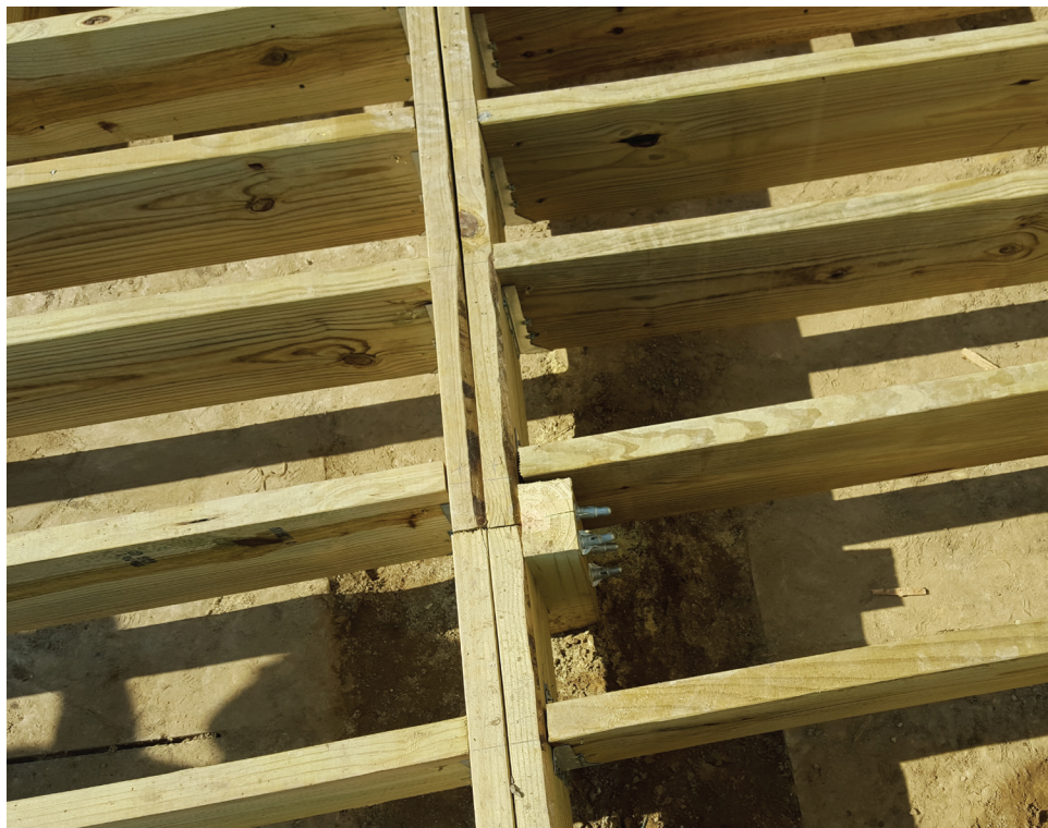
Figure 1. The new deck was built over an old concrete patio. At the bottom of the photo, you can see one of the holes that were cut through the slab in order for us to dig down below frost level and install a proper footing.
