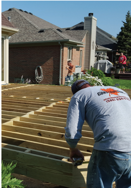
Figure 7. Blocking installed around the perimeter of the frame (left) supports the picture-frame detail used to finish the decking. A contrasting seam board in the middle of the deck highlights the diagonal decking (below). The deck has a tiered fascia detail, which makes the edge of the deck appear narrower (bottom).
