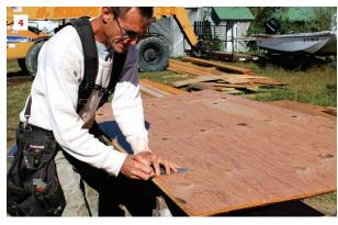
The fastest way to mark sheet goods for cutting is by using a measuring tape with a pencil on the hook end. Move both hands at the same speed for a straight line (1). A T-square makes a good straightedge, but with bumpy edges on the sheets, don't trust it to be square (2). A factory edge from a rip makes a good straightedge for an angled cut (3). To mark a narrow rip, slide a layout square along the edge while holding a pencil at the measurement (4).
