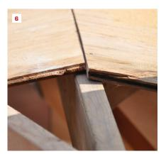
To make a narrow rip without marking a line, clamp locking pliers to the saw table to act as a rip guide (5). Tongue-and-groove edges can make it difficult to make efficient use of angled cutoffs, as when you're working on roofs. Alternating tongue up and tongue down lets you use the same angled cut on adjacent roof planes (6). To avoid confusion while cutting T&G pieces, orient the cutting station to match the direction of the piece as it will be installed.
