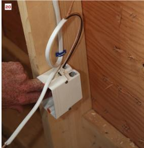
**Receptacle box.** The author's finger gauges where to strip off the outer jacket (18). A utility knife slits the jacket (19). (He adds an inch for slitting the second cable.) Looping cable into the box (20) provides extra cable in case of damage during drywalling.
