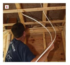
**Drilling and fishing.** The author drills a <sup>3</sup>/<sub>4</sub>-inch-diameter hole (big enough for a maximum of two cables) through the plates and into a joist bay (5). A spooler keeps the cable straight and flat as it comes off the roll (6). The author feeds a length of cable through a joist bay (7) and then loops it as he feeds it into the drilled hole, to keep the cable flat and without a twist (8).
