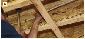
Stapling 101. To staple a run of cable to the side of a joist, the author hooks the cable with one finger and flattens the cable against the joist with the side of his hand (9). While holding the cable flat, he drives a cable staple about three-quarters of the way in (10). Then he reaches over and pulls the cable tight while he finishes driving the staple into the joist (11).
