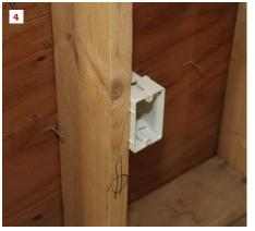
**Getting started.** Before running cable, the author marks the switch locations and notes what each switch will control (1). A circle with two vertical lines indicates a receptacle location (2). The crew installs receptacle boxes using a laser level to keep the boxes at a consistent height (3). Small plastic nubs on the side of the box align it at the proper depth for the drywall (4).
