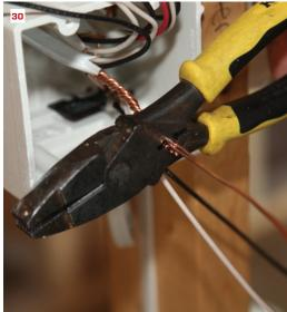
Ground connection. After twisting the ground wires together from all five cables, the author cuts back all but two of the conductors—one for each of the switches. A crimp sleeve large enough for the entire bundle then slips over the twisted wires (29). A special crimping jaw on the pliers collapses and tightens the sleeve to secure the grounds together (30).
