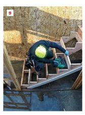
**Wall finish.** If the walls are drywall only, a 1-by nailed to the stringer provides space for the drywall to slide in (5). If a finish skirt will be added, the author nails on a 2-by (6). Risers. Two-by risers provide nailing for each tread. The author starts by applying adhesive to the stringer edges (7), nails on a riser at the bottom and midspan (8), then nails on the remaining risers (9).
