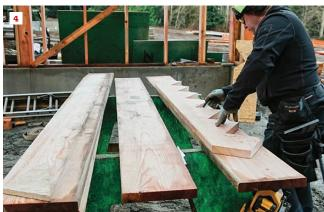
**Cutting stringers.** The most important thing to remember is that all the stringers must be identical. The author lays out the first stringer with a rise and run block (1), then cuts each step with a circular saw (2). He is careful not to overcut, finishing each step with a jigsaw (3). To keep stringers consistent, he uses the first stringer to lay out the second (4) ... and (not shown) the third.
