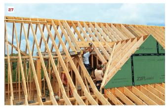
Pairs of rafters straighten and support the ridge. If the ridge needs to be tweaked in the opposite direction, the opposite side goes in first (24). The last of the rafters goes in, leaving the ridge nice and straight (25). The author removes the temporary strips on top of the ridge, leaving a space for ridge ventilation (26). The intersecting gable dormers complete the roof framing (27).
