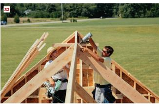
There were no common rafters at the center of this house, so the crew supported the center with a temporary post and braced it back to take the bow out of the ridge (20). The low ends of the rafters were secured first (21), and then the top of the rafter on one side was attached (22). The author toenailed the opposite side so that it could be driven into place to straighten the ridge (23).
