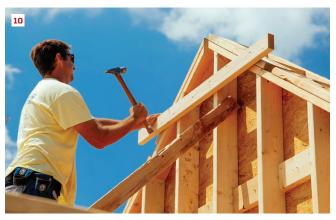
The crew attached a ripping of 2-by stock to the top of the ridge for setting the height of the rafters (7). Strong aluminum staging provided a good working platform for the crew (8). To set the height of a supporting ledger, the author set a scrap of the ridge stock into the slot on the gable (9). The ridge would be nailed to the rake plates at that height (10).
