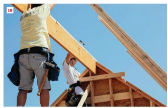
The crew pulled the ridge back so that one crew member could shoulder the end of the ridge onto the ledger (16). They then pushed the ridge into the gable slot (17). At the other end, they had to lift the ridge to drop it into the slot from above (18). One of the crew tapped the ridge down into place (19).
