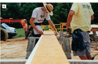
To find the length of the ridge, the author measured to the outside of the wall framing (1). The crew member at the other end of the tape held it at 1 foot for the measurement (2) and did the same when measuring the ridge stock (3). The crew laid out the rafters on one side (4), squared the layout around the edge (5), and then transferred the layout to the opposite side (6).
