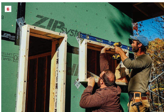
Concrete “cookies” used to brace the wall framing were only partially effective (4). Kelly taped the sheathing joints at openings (5) before screwing on window bucks (6).
