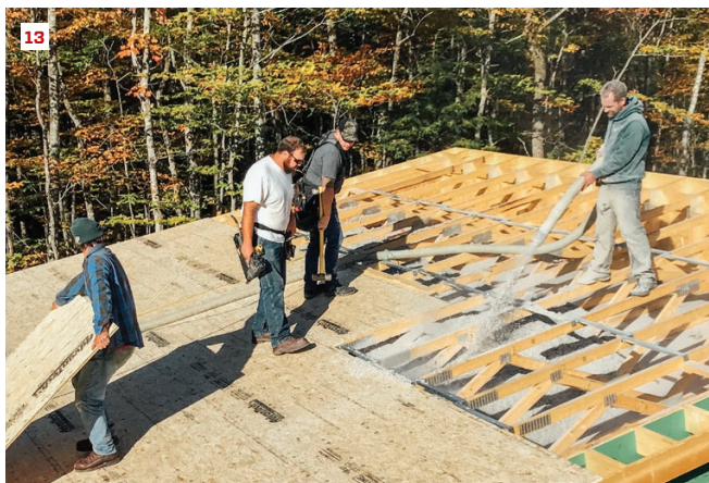
The high-performance roof proved economical. Setting the monopitch trusses (11), installing the OSB air barrier (12), and insulating from above (13) all went quickly.
