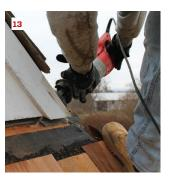
A long blade cuts the nails behind the shingles so the shingles can be removed (11). Here, a special pruning blade turns a recip saw into a landscaping tool (12). The flashing behind this rake trim needed to be replaced; a recip saw clips the nails that were holding the original flashing in place (13).
