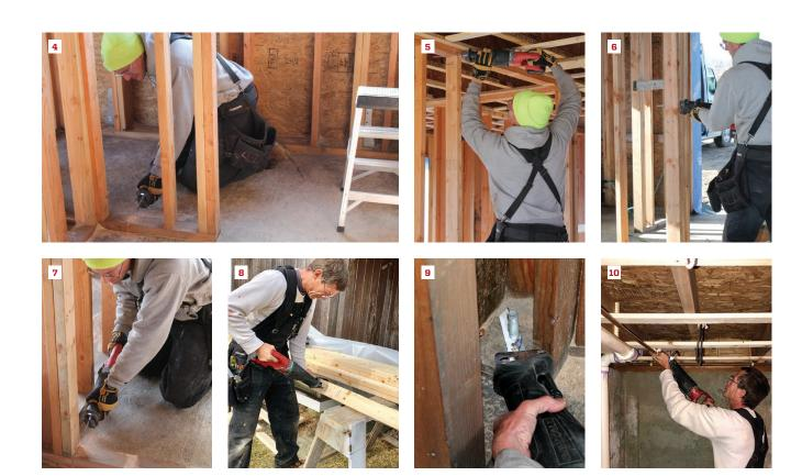
The author slices through a plate to shorten a wall (4). A recip saw makes quick work of removing a stud without damaging it (5). Using wedges to hold the boards apart, the author clips nails to remove a jack stud (6). A recip saw can also cut out a rough sill (7) and make a notch in a stud (8). A metal-cutting blade can slice off a bolt (9), or cut through pipe quickly (10).
