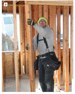
The reciprocating saw on the right in the photo is a corded version from the 1980s, and the cordless saw on the left is much newer and comes with a quick bladechange mechanism (1). An assortment of blades can also be seen in the saw cases. A recip saw can be used to clip the nails at the top and bottom of the studs (2) so a framed opening can be removed in one piece (3).
