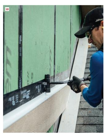
**Ribbon boards** serve as a visual element that helps define gable ends. Here, the author packs out a trim board with OSB ripped narrower than SmartSide Trim boards so the bottom edge of the ribbon overlaps and protects the siding board below it **(8)**. The top of the ribbon needs a Z-flashing **(9)**, which must be integrated with the Zip System WRB, using Zip Tape. Like all adhesive flashings, this needs to be rolled to ensure a tight, lasting bond **(10)**.
