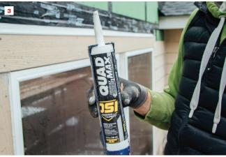
**Sealing cuts.** All cuts, rips, and end cuts need to be sealed. If the siding boards are acclimated, the author hits the edges with spray-on primer, such as Zinsser Bulls Eye 1-2-3 Plus (1). If the wood needs to acclimate, or if the weather is wet, the author will install the siding first and caulk the gaps later (2). LP's instructions call for an ASTM-C90 minimum Class 25 sealant; the author uses OSI's Quad Max (3).
