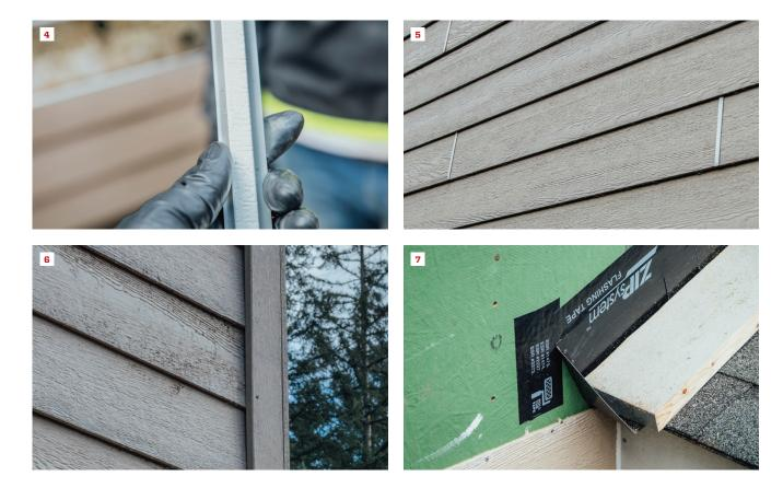
**Devil's in the details.** SmartSide can move and squeeze out caulk at butt joints. To avoid this, seal the butt joints with H-Moldings (4). These are still noticeable, but vastly better looking and more durable than ridge lines of caulk (5). At corners, the author prefers "spider catcher" downboards, which protect the siding ends (6). Kickout flashings are a must; a 2-by on the roof is used to butt siding pieces to create a  $1^1/2$ -inch gap at the roofline (7).
