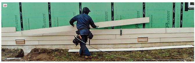
**Helpful jigs.** The author depends on two jigs made PacTool. The Gable Slide easily adjusts to the rake angle of the gable end (11). Here he's using it to find the angle for the last piece of the ribbon board (12), but that same angle will be used for all the siding that fills in the gable end, as well. The Gecko Gauge, to the right of the author in the photo (13), holds a long run, making it easy for one person to install long lengths of siding.
