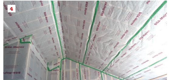
Early adopters are starting to try out Siga Majrex in projects such as these cathedral ceilings, constructed for high-performance homes in British Columbia (3) and Maine (4) .
