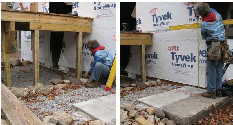
Figure 1. A dropped 2x6 header fastened to support posts provides a solid attachment point for the stairs (above left). Rise and run—and therefore the size of the risers and treads—is determined by marking a level line from the top of the decking, and then measuring out from the front edge of the decking and up from the end point of the stairs on the landing (above right).
