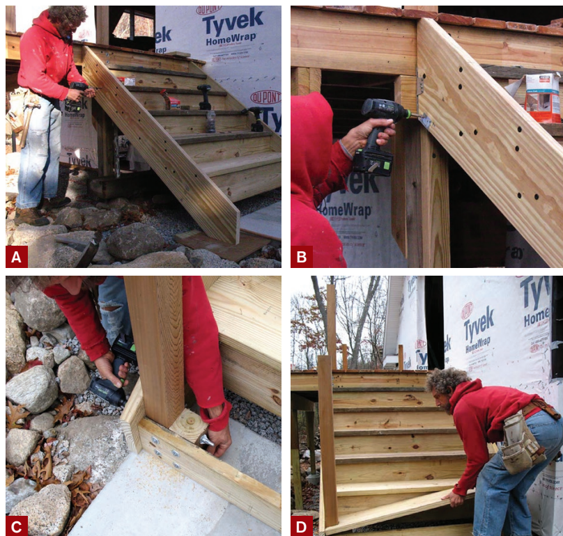
Figure 5. Flat-head structural screws driven through pilot holes in the stringers and into the treads and risers draw the assembly together (A). After the author slides the stairs over into position, he uses stair-stringer connectors to hang the stairs from the rim board and 2-by header (B). ThruLok screws and a hefty blocking detail fasten the guard post to the stringer and the structural riser (C). The final tread is notched to fit around the post, then fastened in place with structural screws (D).
