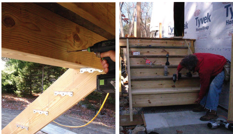
Figure 4. Five-inch-long structural screws driven through the risers into the back edge of the treads 12-inches on-center reinforce the treads (above left). The front edge of the treads and the top edges of the risers are also fastened together with long structural screws (above right).
