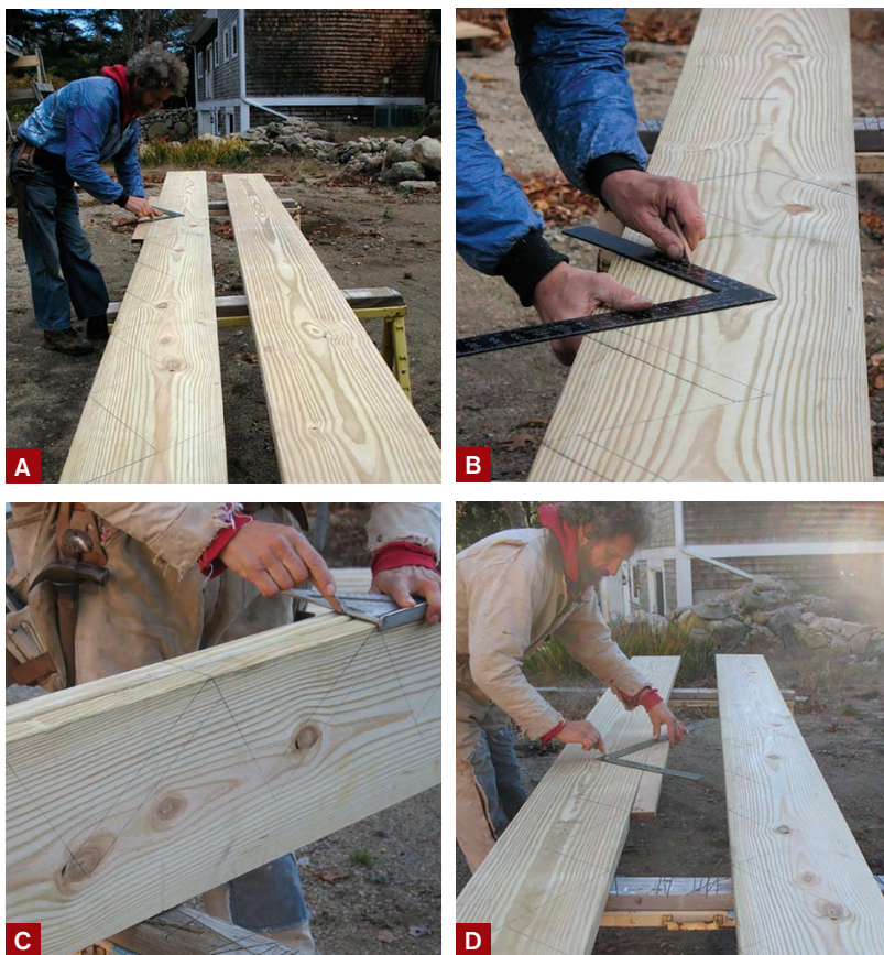
Figure 2. For laying out treads and risers on a pattern stringer, a 1-by straightedge screwed to a framing square provides more accuracy than stair gauges (A). To locate the metal stair brackets, mark both the tops and bottoms of the treads (B). Tilt the two stringers on edge to transfer the tread-riser intersection to the other stringer (C), then lay out the remaining stringer so that it is a mirror image of the pattern (D).
