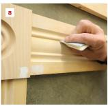
**Hand sanding.** Hand sanding leaves more dust, but it is the best way to sand details such as the circles in a rosette (6). Slightly breaking the sharp edges of the trim helps with paint adhesion, and hand sanding is best for this task (7). Folding sandpaper to a sharp crease can be effective for smoothing out the narrow grooves of a trim profile (8).
