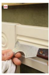
**Detail caulking.** A painter's 5-in-1 tool becomes a handy putty knife for caulking hard-to-reach detail areas around the molding. For flat, or square, surfaces, the square edge of the tool works well to fill the joint **(22)**. For tight and narrow areas such as the groove on this molding profile, the pointed end of the 5-in-1 tool works best for tooling the caulked joint **(23)**.
