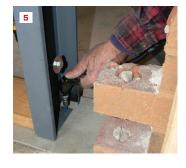
The author opens up a window opening for the door (1) and then forms a new sill (2). Bolts threaded onto the jambs form masonry anchors for the side jambs (3). To anchor jambs to the sill, he drills holes (4) and then drives Tapcon concrete anchors into the holes with a flexible drill (5).
