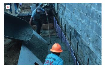
Masons apply brick veneer to the two-story block addition (1). An existing 8x10 bump-out addition was removed prior to construction (2). During demolition, it was discovered that an abutting neighbor's two-story addition was built on undersized footings (3). New footings had to be poured with concrete wheelbarrowed through the house from a mixer truck parked street-side (4).
