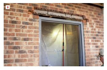
Braces clamped to the frame and attached to the joists hold the door frame in place (6). Spreaders keep the jambs from bulging inward while the brickwork and grouting is completed (7). Bricks fill the toothed-out sections near the bottom of the opening (8), and bricks at the top corners of the frame bring the masonry to a height 1/2 inch above the header jamb (9).
