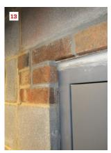
The author grouts the jamb channels from the top, scraping the mix into the header channel and pushing it into the sides (10). After filling the head channel about two-thirds of the way, he embeds rebar in the mix (11), then finishes grouting (12). Steel lintels (seen above the door) sit on top of the corner bricks and support the brickwork on both sides of the door (13).
