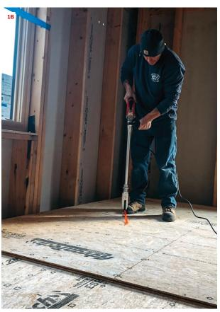
The crew installed the second layer of subflooring perpendicular to the first with joints staggered in both directions (15). They made sure to maintain 1/8-inch clearance between the sheets on all sides. After tacking the sheets in place, one crew member screwed the subfloor layers together with an auto-feed screw gun (16). At the doorways, they held the top layer of sheathing back 5 inches. Flexible flashing tape laps onto the second layer of subfloor, forming a sill pan for each door (17).
