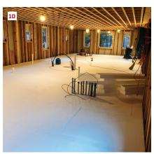
After the building had been dried in, the crew put down sheets of 4-inch EPS rigid foam insulation over the slab (6). The insulation had to be cut out around all plumbing stub-ups through the slab (7). In a few places, the crew notched out the insulation to reposition some of the services (8). They also cut out around structural columns that supported a space between sections of the house (9). Clear-span trusses allowed the entire floor to be done without dealing with interior partitions (10).
