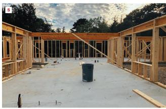
As this was a slab-on-grade system, all of the utilities and services had to be in place before the slab was poured (1). The next step was laying down and compacting a layer of crushed stone (2). To help control moisture, the crew put down a layer of 10-mil polyethylene sheeting—which also acted as part of the air barrier—over the crushed stone (3). The slab was placed in the usual fashion over the poly (4), and the framing crew built and raised the exterior walls to support the truss roof (5).
