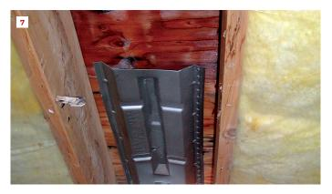
**Poor air control.** Each of these show vent channels that are supposed to be directing outside cold, dry air from the soffit to the ridge, but because there is no continuous air control layer in the ceiling plane, the vents are directing leaking warm, moist air up against the cold underside of the roof sheathing.
