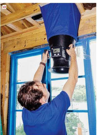
The Alnor flow hood measures airflow through a supply register. Because he's testing the system with no drywall installed, Harris masks off the parts of the flow hood that would ordinarily be blocked by the drywall (11, 12). Then, with the Duct Blaster fan set to supply the design airflow for the system, he checks the output of every register in the rooms served by this duct run (13), to make sure that the actual flows match the design values for the system.
