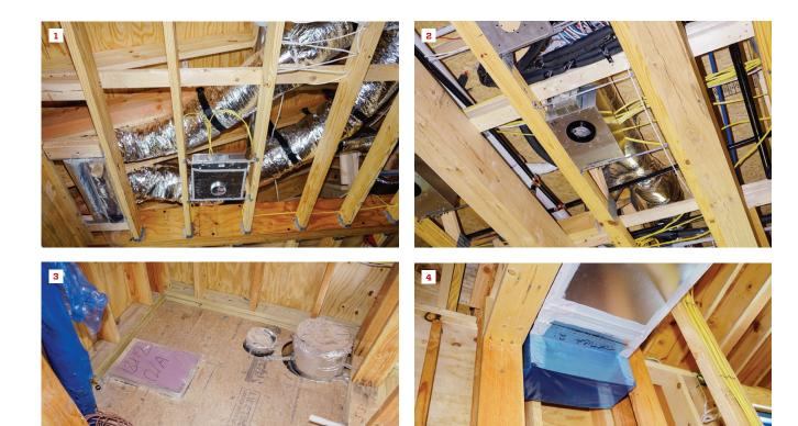
Ductwork installed in this high-end custom home under construction will be difficult to access after the ceilings are drywalled (1, 2). At this point in the job, however, the air handlers have not been installed. Instead, supply and return duct runs are capped with plastic wrap and tape in the mechanical room (3, 4). Positive Energy duct expert Sean Harris will test the duct system now, and then return later in the job to re-test the fully assembled system.
