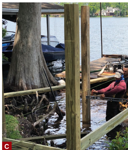
Figure 1. A water jet is used to set 6x6 PT pilings into the lake bottom (A). Then 2x8 stringers are nailed to pilings a minimum distance above the water level, per state and local codes (B). A second set of pilings are set parallel to the first (C). The crew sets a maximum of seven or eight pilings per side, then starts to frame the structure to stabilize them (D).
