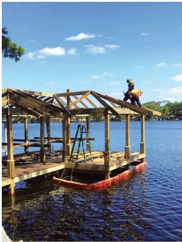
Figure 5. When the crew is working over water, care must be taken to collect offcuts. The orange turbidity curtain is a requirement for containing construction debris.
