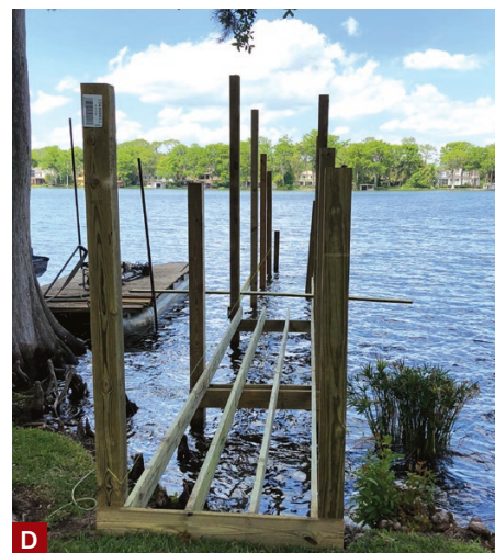
Figure 1. A water jet is used to set 6x6 PT pilings into the lake bottom (A). Then 2x8 stringers are nailed to pilings a minimum distance above the water level, per state and local codes (B). A second set of pilings are set parallel to the first (C). The crew sets a maximum of seven or eight pilings per side, then starts to frame the structure to stabilize them (D).
