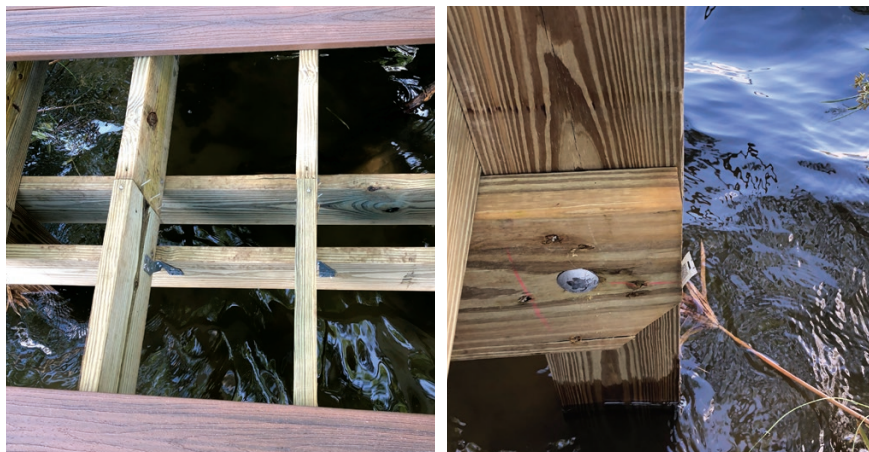
Figure 2. Hurricane clips tie the intermediate stringers to the 2x8 cross beams (far left), while 10-inch-long-by-5/8-inch-diameter HDG through-bolts fasten the cross beams to the pilings (left).
