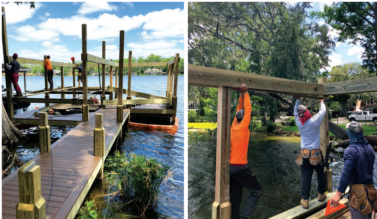
Figure 4. When plans include a boathouse or other roofed structure, the crew installs longer pilings to support the framing (above left). To create the box beams that support the roof, the crew fastens 2x10s to the inner and outer faces of the pilings, then fills the gap between the 2x10s with a 2x6 filler, making a convenient wiring chase (above right).
