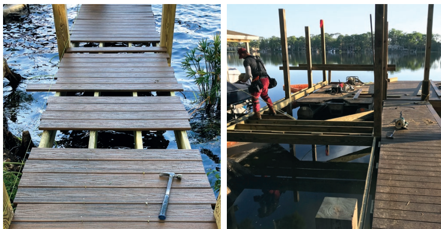
Figure 3. The crew dry-lays the decking to check the layout, spacing the deck boards with 16d nails to make sure water will drain off the dock quickly (far left). To provide support for a picture-frame border, the crew installs extra stringers between the pilings and adds blocking (left).
