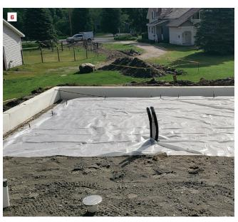
**Prepping for the slab.** After putting down horizontal wings of insulation around the base of the forms, the excavator backfills around the forms to lock them in place. Soil added inside the forms is compacted (5), and then the crew spreads a layer of poly as a vapor barrier below the concrete slab (6). Vertical sections of rebar will tie into the rebar grid for the slab.
