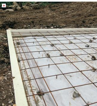
**Rebar grid.** A grid made from ½-inch rebar forms the reinforcement layer for the monolithic slab (7). The ends of the bar insert into the foam, and pieces of CMU act as chairs for the grid to sit on. Each intersection is wire-tied together and anchored to the vertical rebar sections. An additional layer of rebar below the main layer reinforces the built-up edge of the slab (8).
