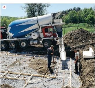
**Excavation and footing.** The first step is excavating for the foundation assembly. With the excavation open, the crew can put down a layer of crushed stone. The crew sets up 2x4 forms for the footing, using a laser to make sure that they are perfectly level (1). After the crew stakes the forms in place, a concrete truck carefully fills them (2).
