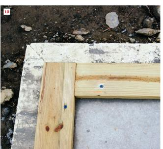
**Slab placement.** The concrete crew places the slab, screeding the mix flush with the top of the forms (9). The treated sills for the walls attach to the slab with concrete screws for positioning (10). Embedded J-bolts around the perimeter of the slab provide permanent anchoring for the framing.
