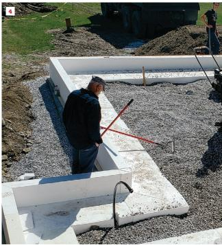
**Insulated forms.** After the footings set, the crew cuts and fits insulated forms made from EPS foam for the slab (3). The forms cut easily with a handsaw, and the crew miters the corners. Next, they even out the ground inside the forms with a fresh layer of crushed stone, compacting the layers as they go (4).
