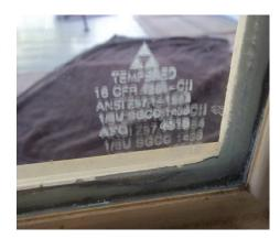
Tempered-glass etching. This etching (shown several times its actual size) on the corner of a glass panel indicates that the glass is tempered. Tempered glass is stronger than conventional plate glass and is used in situations where stronger glass is required, such as for windows at the bottom of a staircase or in a bathroom where a wet floor can be a walking hazard.
