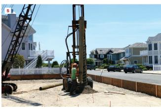
**Piles in the ground.** Before pilings are driven, an engineer lays out the positions of each one (1). A dump truck delivers the pilings (2), the length and diameter of which are based on the soil requirements. A long auger digs a hole at each location (3). A crew member fastens a loop of chain around each piling (4), and the crane lifts the piling and swings it to the hole. The crew member then guides the piling into the hole (5) and levels the ground around the piling with a shovel.
