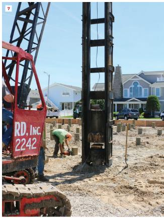
**Pounding the pilings.** When all the pilings are in their holes, the crew attaches a sled with a 1-ton driving hammer to the crane. The crane positions the sled over each piling and a crew member marks 6-inch increments on the sled to monitor how deep the piling travels with each hit (6). The crane raises the hammer and drops it on the piling (7), while the engineer (slightly out of the photo) witnesses and records each piling.
