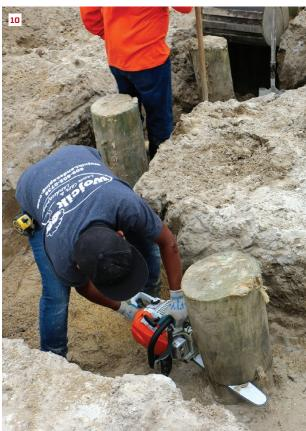
**Digging for the grade beam.** A mini-excavator roughs out the trenches, digging between the pilings **(8)**. The crew follows, evening out the floor of the trench with shovels to prep for the concrete **(9)**. The crew keeps the depth of the trenches consistent using a laser level. As the trenches are finished, one crew member cuts the pilings 4 to 6 inches above the floor of the trench with a chain saw **(10)**.
