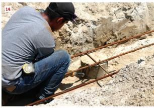
**Grade beam reinforcement.** The crew installs #5 rebar to reinforce the grade beam. The first pieces are short lengths of rebar that rest on each piling (11). Next, three lengths of rebar sit atop the short pieces (12). Where two or more lengths are needed for a straight run, the pieces overlap and are tied together. At intersections, the rebar from one trench sits on top of the other and they are tied together (13). Finally, the crew bolts S-hooks to each piling to anchor the rebar (14).
