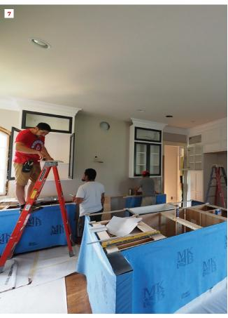
The difference in crown angle can be seen between the wall cabinet in the foreground and the one in the background (6). But when viewed from across the room, the difference is hardly noticeable (7). Slight variations in the ceiling can often be remedied by floating drywall compound down to the level of the crown molding (8).
