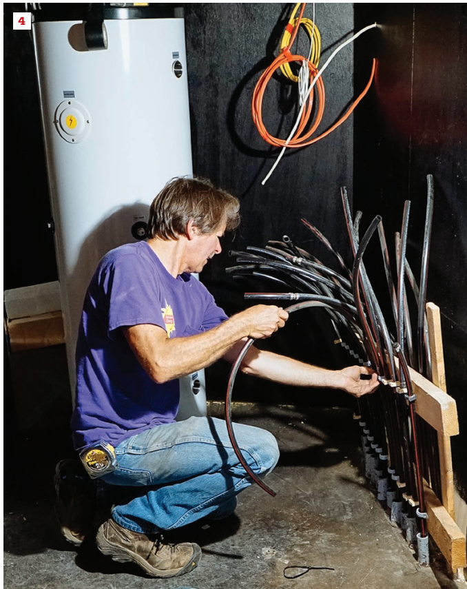
Radiant floors team with hydro-air. ReVision Energy's Chris Blaisdell works on the hydronic tubing for a radiant slab in a custom house (4). Behind Blaisdell is the hydronic buffer tank for the system. On the second floor of this home, a SpacePak high-velocity hydro-air unit (5) will supply heated or cooled air using fluid supplied by the same outdoor-mounted heat pump.
