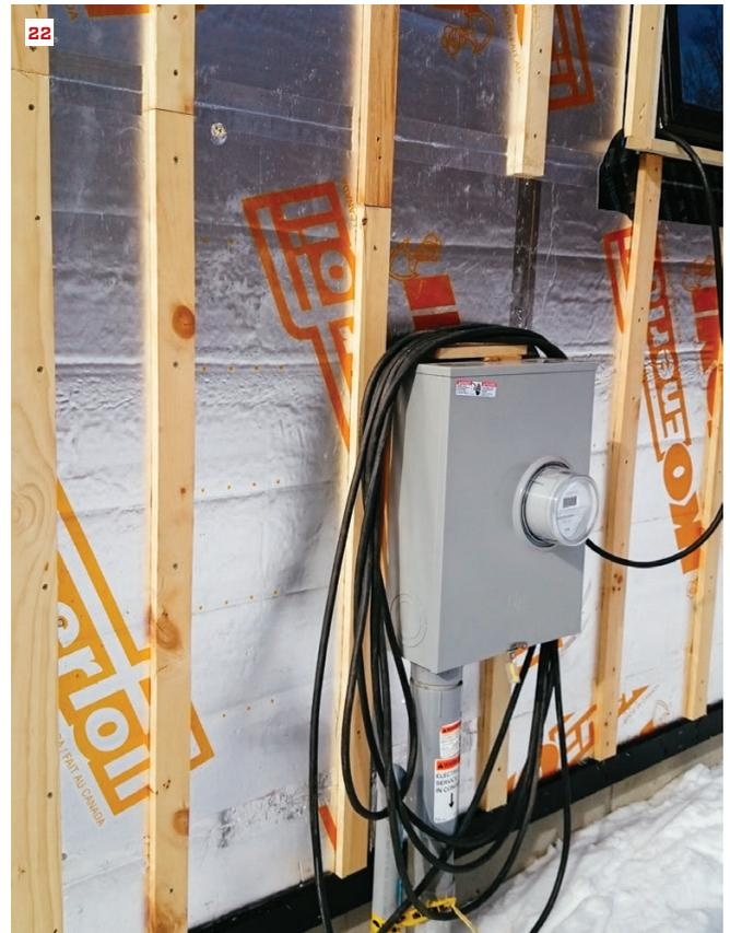
A carpenter scribes a board around a window in an open rainscreen system, with spacing between the boards and a space left under the window sill (19). A temporary strip creates the open space at a corner board (20). Furring strips end well above the head flashing over a window (21). Services such as this electrical meter are furred off the wall as part of the siding (22).
