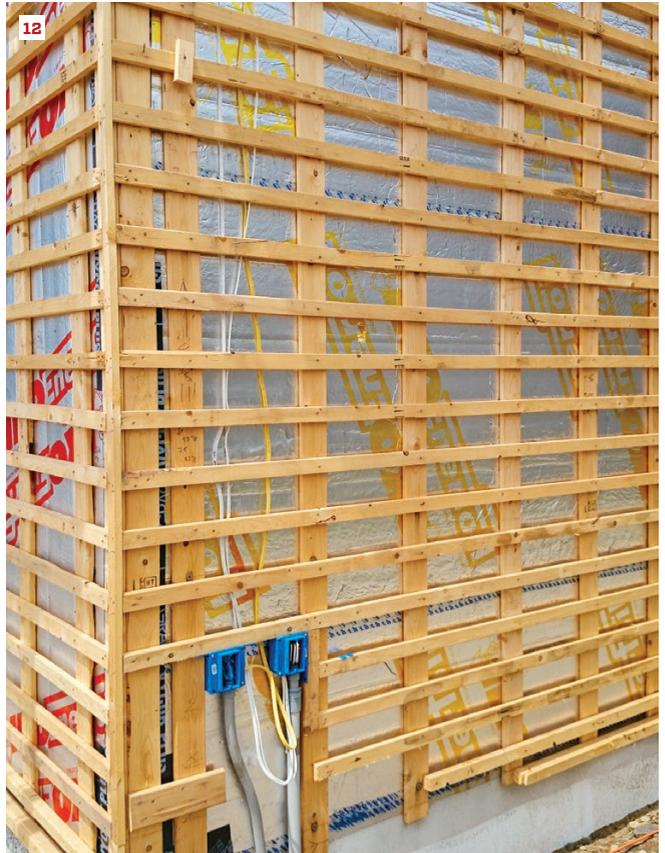
A second horizontal layer of furring provides nailing for vertically applied siding, such as this corrugated metal (10). If there isn't enough depth for the second layer of furring, the strips can be installed diagonally with breaks to allow water to drain down and out of the bottom (11). Site-built rainscreens can be used for shingle siding, but this application is labor intensive (12).
