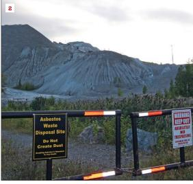
Asbestos fiber is loaded into 100-lb. bags at Ruberoid Co.'s Vermont mine, circa 1950 (1). The Eden-Lowell mine was the first (and largest) commercial asbestos mine in the U.S. Thirty million tons of tailings, upwards of 350 feet high, were left at this 1,550-acre site (2). Trucking the tailings off site as well as turning the mine into a solar farm have been proposed.
