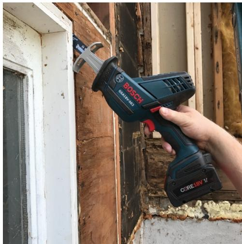
The rounded footplate of the Bosch made cutting much smoother with the blade buried into the work.
