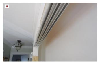
The author uses a track saw to remove a 6-inch-wide section of flooring for the guide tracks (5), finishing up near the jambs with a multi-tool (6). Strips of flooring fill the gaps between the tracks, which are screwed to the subfloor (7). The author screwed the overhead tracks through the jambs and into the header in positions dictated by manufacturer's instructions (8).
