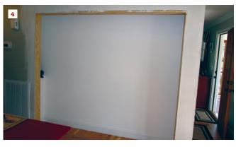
This pantry had three inconvenient outswing doors. Here, the doors and an intermediate post have been removed (1). Having taken out the existing headers (2), the author screws a single 9-by-5<sup>1</sup>/4-inch U-shaped header to the top plate (3). To accommodate the three bypass doors, the new 53/4-inch-wide finish jambs are wider than the existing 2x4 walls, and they are flush with the drywall on the outside of the pantry (4).
