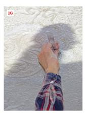
After the damaged piece has been removed (11), Ron applies a bonding agent over the old, dusty lath (12), then spreads a thin coat of plaster (heavy on the gauging, light on the lime) to the repair area (13). Squeeze-out from the replacement piece is tooled around the edge (14). Finally, touch-up lime putty is feathered to the existing painted surface, with the excess wiped (15) and tooled (16) off the existing paint.
