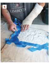
Master plasterer Ron Bisson inspects his replacement plaster flatwork (1), which will be used to repair the main entry hall ceiling of the Fairbanks Mansion in Vermont (2). Prior to making a mold, his son, William, brushes on one of seven coats of flex wax over an intact motif (3). Then the wax impression is removed from the ceiling and prepped for mold making (4).
