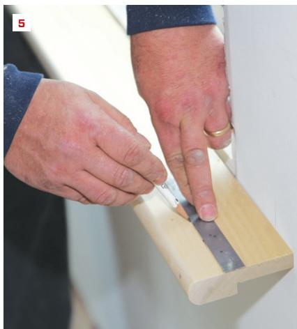
Measuring from the wall, mark that same distance near the end of the horn (4). Draw lines to connect the measurement marks (5). Note that this carpenter stepped the stool to fit tight against the factory jamb, and he drew in that additional line. After installing the stool, he added narrow strips to bring the jambs flush with the drywall for installing the casing.
