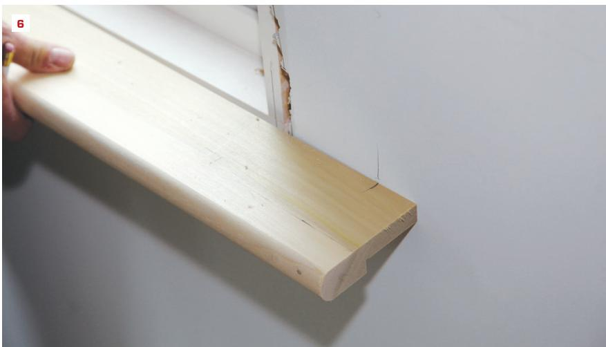
The lines drawn will guide the saw to remove the waste from each end of the stock. Before releasing the stock from the wall, transfer the mark that you'd made earlier on the wall (to indicate the overall length of the stool) to the stock (6). At the opposite side of the window, repeat the entire layout and marking process for the other end of the stool.
