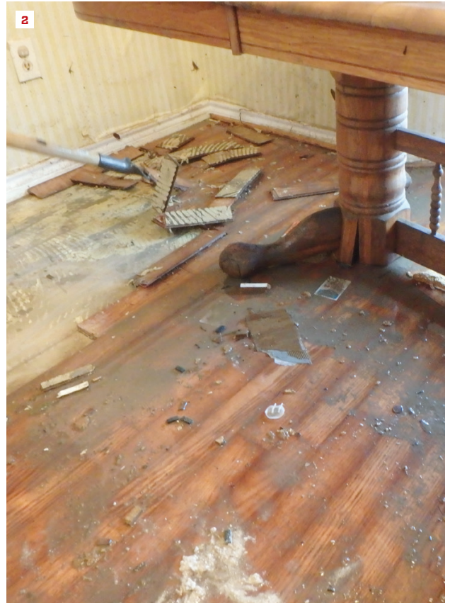
Up to the eyebrows. The author's house, which backs onto a creek in Friendswood, Texas, flooded 5 feet deep in Hurricane Harvey (1). All the interior materials and finishes were ruined, including the wood flooring shown here (2).
