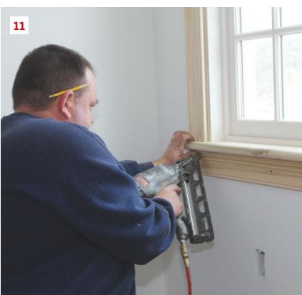
Set the head casing aside and mark the length of the opposite jamb casing (6). Make a 45-degree-angle cut at the top end and cut a slot for a biscuit. Then tack the jamb casing in place on that side (7). The drywall around window openings often sits proud of the jamb extensions. In the photos, the carpenter has removed some of the drywall to allow the casing to lie flat against the jambs. He also drove an additional nail through the outer part of the profile to hold the casing flat.
