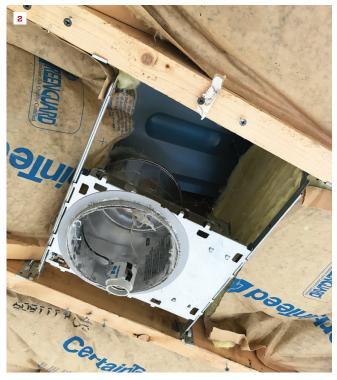
Water stains on the drywall of this cathedral ceiling look like they might have been caused by a roof leak (1). But given the location of the water stains, the author knew this was not a leak, but rather condensation due to poor insulation and air leaks around the recessed light fixtures (2).
