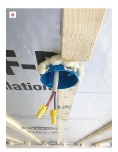
To make it easier to air-seal and insulate the new ceiling, the author assembled light-housing boxes made from foil-faced rigid foam (6). They were tightly taped at all corners and to the continuous layer of rigid foam fastened to the ceiling joists (7). After strapping the ceiling in preparation for drywall, the author sealed all penetrations—including the electrical box for a ceiling fan—with canned foam sealant (8). The new worry-free ceiling is shown at right after the first coat of mud (9).
