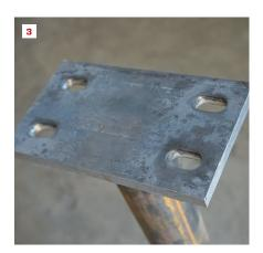
In residential steel work, contractors are likely to encounter steel plate (1) and columns of various shapes (2), shown here in their racks at a metal yard. One example of using the two together is a connection plate welded to a steel column (3).
