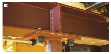
When satisfied that the base plate is tacked square to the column, the fabricator completes the weld along the entire joint (26). Setting the column in a vertical position provides a more comfortable position for the fabricator to weld. The finished weld should have a consistent width, shape, and pattern along its entire length (27). The standard finish for residential steel is red oxide primer (28), an anti-corrosive coating that helps prevent rust.
