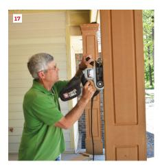
Before setting the second half of the column in place, the author ran beads of glue along the edges (15). He tacked the halves together to align them, then nailed the second half of the column to the horizontal 2x4 blocks he had installed earlier. With the sides joined together with glue and nails, he clamped the assembly together (16). After allowing the glue to set, the author removed the clamps and used a belt sander to smooth the edges (17).
