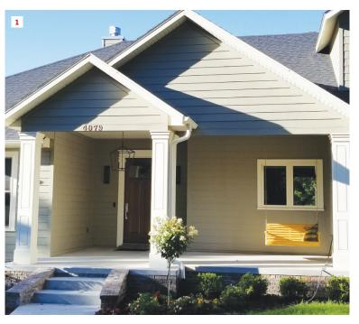
The 4x4 posts that supported this porch looked spindly and out of proportion, so the author and his client decided to wrap the posts with a decorative covering that mimicked raised-panel columns. The author made the columns from exterior-grade MDF and routed the panel detail.
