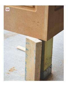
On site, the author began assembling the columns by adding shims to create a plumb surface on each post (11). He fastened the first half of the column to the post with galvanized finish nails (12), holding it at the proper height with a 2x4 spacer block (13). Then he nailed pairs of horizontal 2x4 spacers to the top, middle, and bottom of the post for attaching the second half of the column (14).
