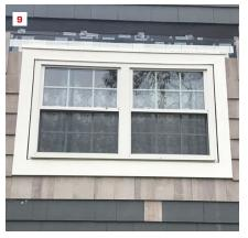
sheathing with flashing tape, and the nails through the flanges were pretty rusty from water getting behind the casing. After pulling the nails and checking behind the flashing to make sure the sheathing hadn't rotted, I renailed the side flanges with 2-inch galvanized roofing nails.
