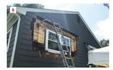
Rot was visible from the ground (1). A closer check revealed the causes: no drip cap over the window casing, and siding caulked to the casing (2). In addition, the flashing tape had been improperly installed (3), and the bottom casing had been caulked to the window (4). Before repairs could proceed, the siding was peeled back (5).
