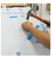
One allowable method for protecting the deck is to install double-coverage asphalt-saturated felt before shingling (3). Fasten the felt to the roof with cap nails, 6 inches on-center at the edges and 12 inches on-center in the field (4). Alternatively, you can seal the sheathing seams using peel-and-stick tape (5, 6) and protect the roof using a synthetic roof underlayment, following manufacturer's instructions (7, 8).
