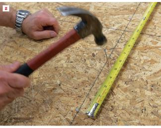
Roof sheathing—either plywood or OSB—should be a minimum of  $^{7}$ /16 inch thick (1). Within 4 feet of the rake, sheathing panels should be nailed to the roof with ring-shank nails spaced 4 inches on-center on the edges and 6 inches on-center in the field (2). On the rest of the roof, the ring-shank nails should be spaced 6 inches on-center everywhere.
