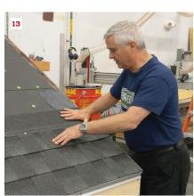
A good weather seal between shingles and underlayment is key to preventing damage in a storm. One approach is to apply a self-adhered manufactured starter strip (9). Another option is to embed the starter shingles in a ½-inchthick bed of roof mastic (10, 11). You can also use this approach for sealing shingles along the rake (12, 13).
